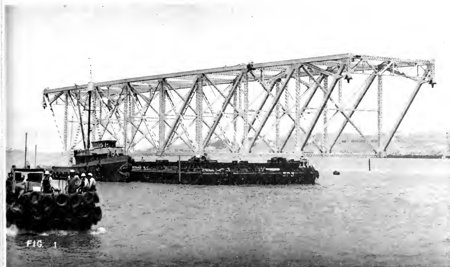
Aluminum falsework truss being towed to bridge
